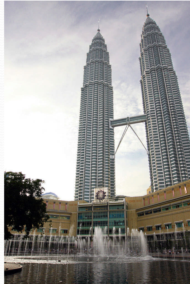
Headquarters at the PETRONAS Twin Towers
